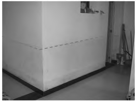
图6 东界脑村居民家里清晰的淹没线 Fig. 6 Clear flood line in a resident's home
