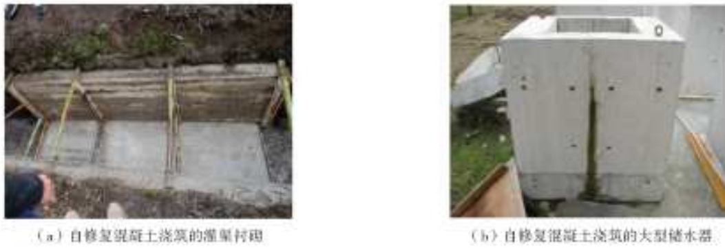
图 3 (a) 自修复混凝土浇筑的灌渠衬砌 [83] , (b) 自修复混凝土浇筑的大型储水器 [84] Fig. 3 (a) Canal lining built with self-healing concrete [83] , (b) Large water reservoir built with self-healing concrete [84]
