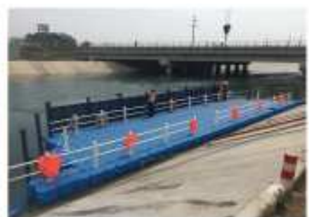
(c) 挡水面板安装
